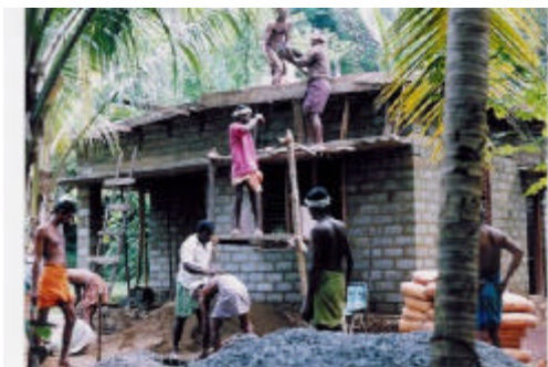
House No 30 under construction last year
